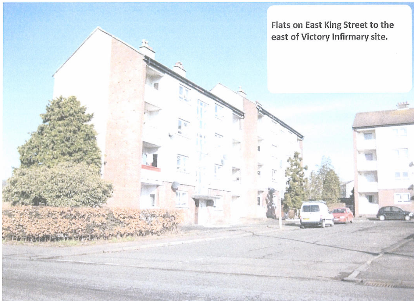
Ex local authority flats on East King Street, opposite the front of the Victoria Infirmary site.
